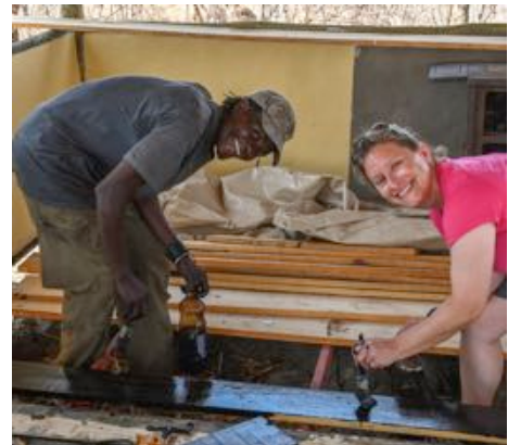
Jennifer from OKC assisting MK with construction of dining area
